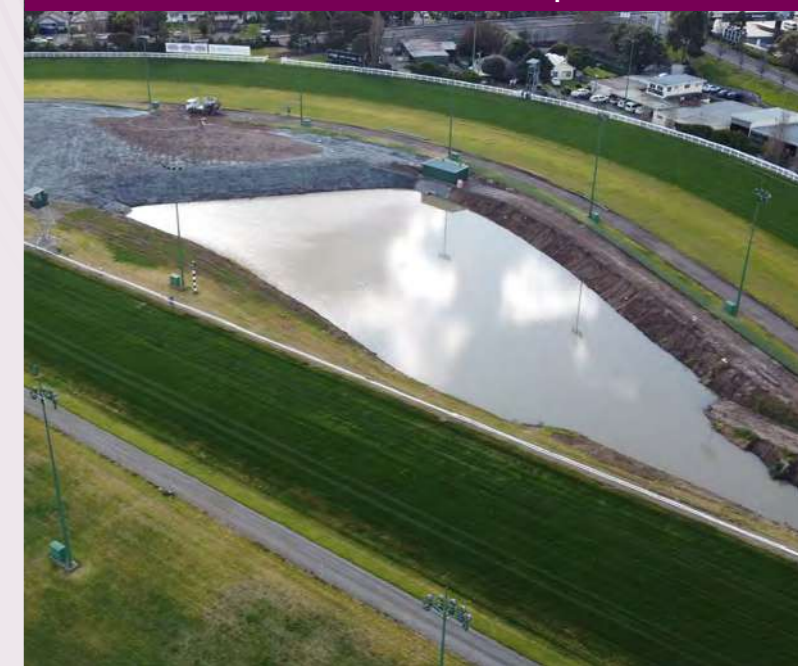
DAM consolidation on the infield completed
